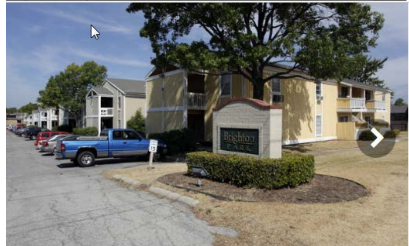
Brighton Park Apartments
